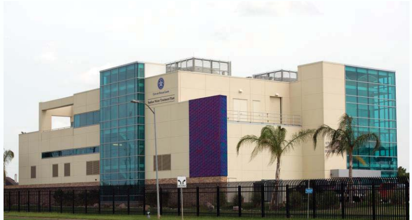
Figure 1-4. Photograph of the Surface Water Treatment Plant
