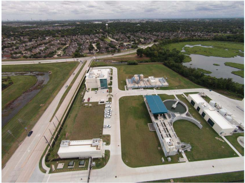
Figure 7-2. Photograph of SWTP (Aerial View)
