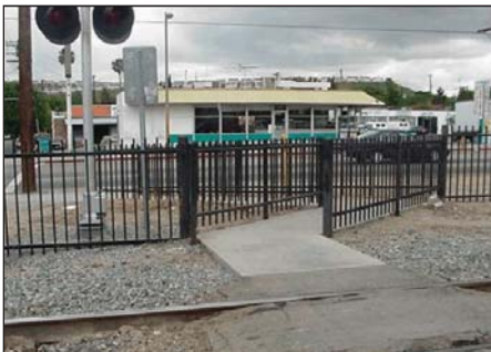
Figure 3-40 Examples of pedestrian warning signals at railroad crossings. Image source: Federal Railroad Administration
