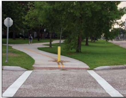
Figure 3-30 Diverters causing bicyclists to slow down.
