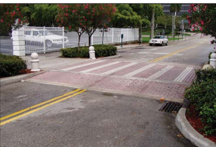
Figure 3-27 Raised crosswalk. Source: Dan Burden - pedbikeimages.org
