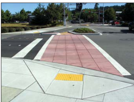
Figure 3-6 Painted crosswalk. Source: Dan Burden - pedbikeimages.org
