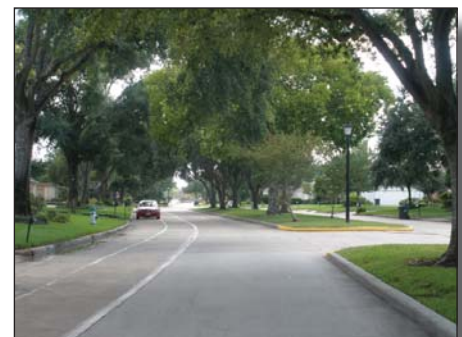
Figure 3-14 Existing bicycle lane adjacent to on-street parking in Sugar Land (along Country Club Blvd.)
