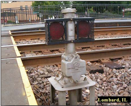
Figure 3-40 Examples of pedestrian warning signals at railroad crossings. Image source: Federal Railroad Administration
