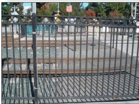
Figure 3-41 Examples of fencing at railroad crossings. Image source: Federal Railroad Administration
